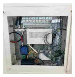
To activate the data outlets in your house, all you need to do is plug the Ethernet cables to the data points in your open networks box, as shown on the left.
