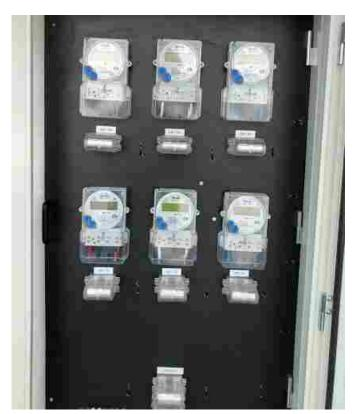
The mains for each townhouse will run from this metering panel, through a penetration in the podium onto cable tray fixed to the soffit of the podium, and up into the main switch located in the switchboard for each respective townhouse.
