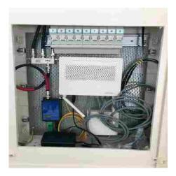
The image on the left shows the inside of your open networks box located in your garage. There are 9 data points which you can see at the top of the box. These data points run to outlets throughout the townhouse.
