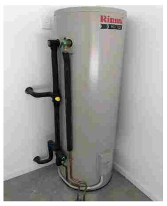
The image on the left shows the Rinnai 160 Litre Hot water storage tank that will be located in your garage or under the stair area. It is hardwired on its own circuit, which can be isolated at the switchboard, and easily accessible for any maintenance in the future.
